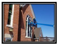
sure to take some time to look at the repairs made to the outside of the stained glass windows. The work included the removal of the old storm windows, a "re-cementing" of the outside glass which deep cleaned the stained glass and adhered the lead to the glass, frame repair, caulk paint, and Lucite/aluminum а new
